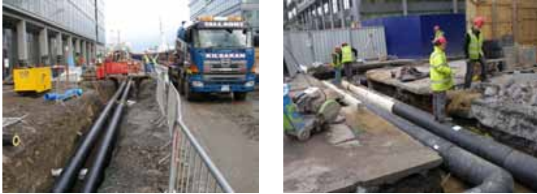
Figure 2: Installation of District Heating Pipes at Spencer Dock
