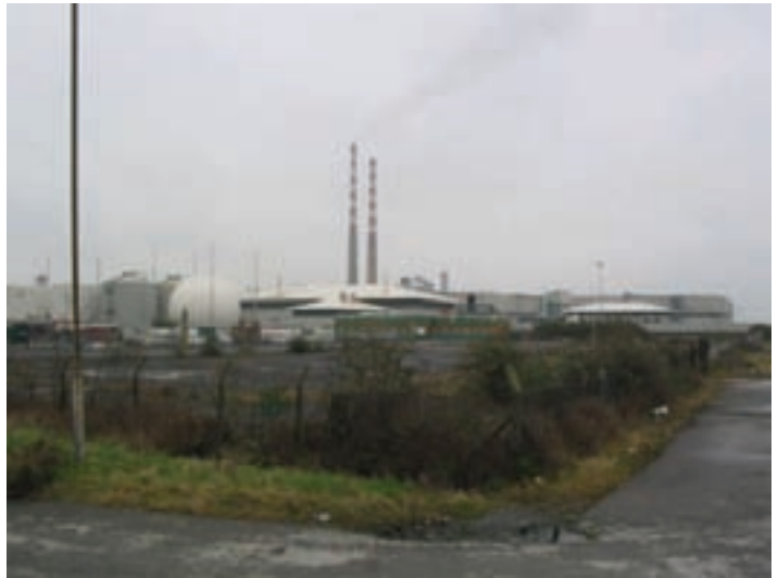
View from the south-western corner of the site with the twin Poolbeg stacks in the background
