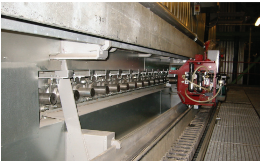
Figure A5.5 Mechanical rapping device at Elsam's Odense Waste to Energy Facility
