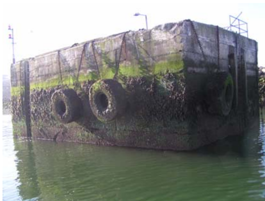
Plate 5.15 The structure of site Lb.
