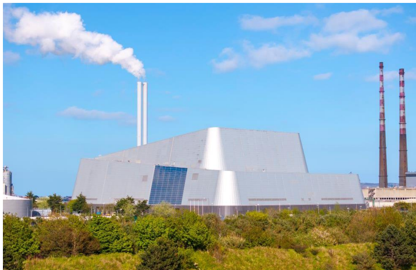
Emissions from the Dublin Waste to Energy facility are rigorously monitored
